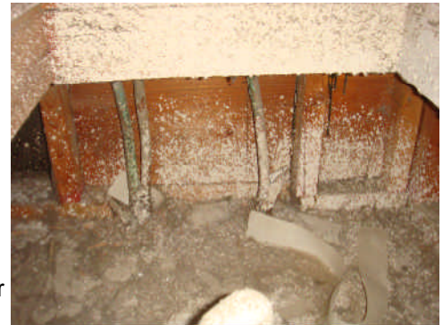
Insulation is covering plenum & ducts.
