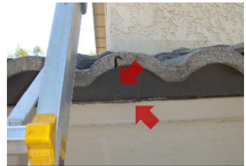
Crushed pan flashing & no opening.
