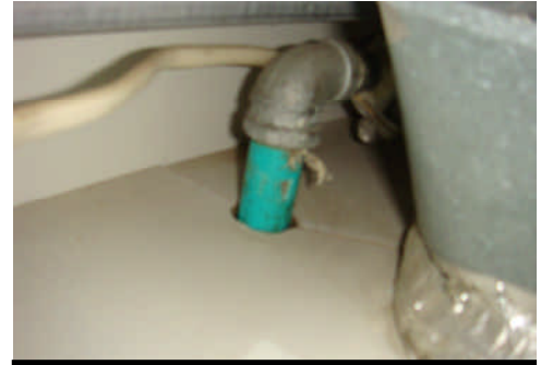
Gas pipe below the cooktop cabinet shelf.
