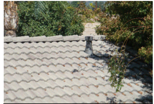
Cut the tree back from the furnace flue.
