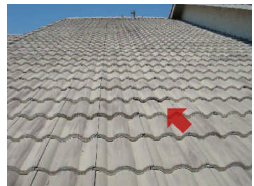
Right side tile visible fasteners.
