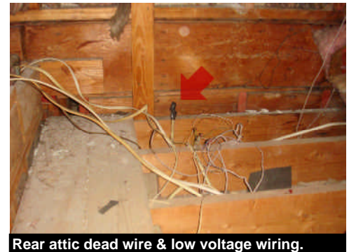
Rear attic dead wire & low voltage wiring.
