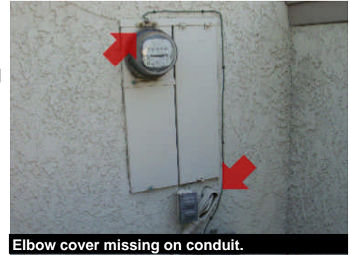
Elbow cover missing on conduit.
