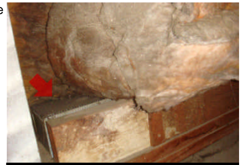
Original combustion air opening blocked.
