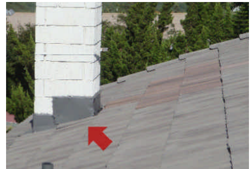
Uneven tile should be evaluated.
