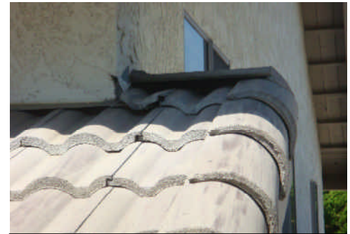
Irregular tile installation at the rear.
