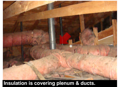
Insulation is covering plenum & ducts.
