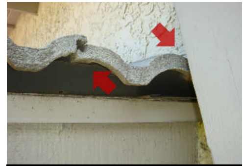
Tile & riser has an irregular fit.
