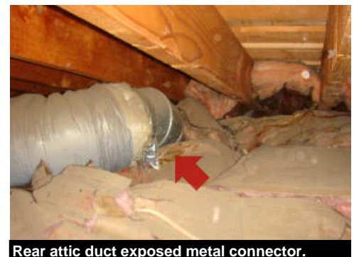
Rear attic duct exposed metal connector.
